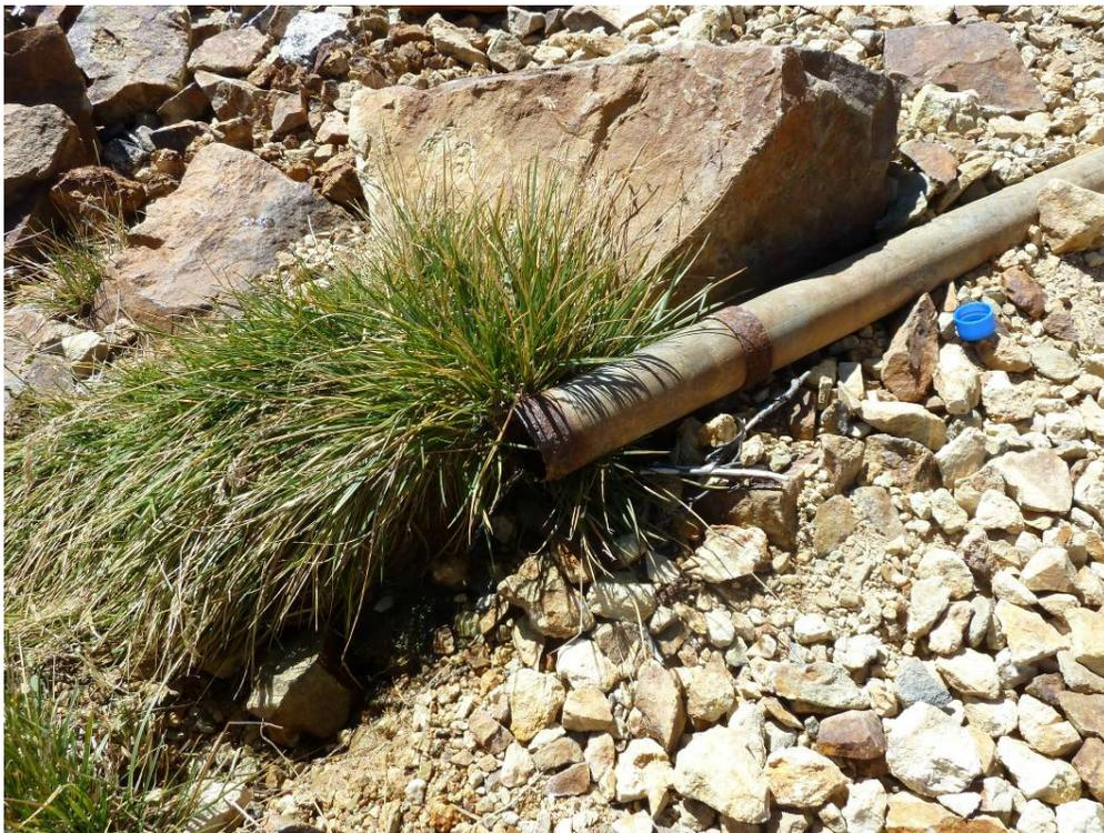
*Photograph 12b: Pipe draining the upper Mary Ann Mine collapsed adit.*
