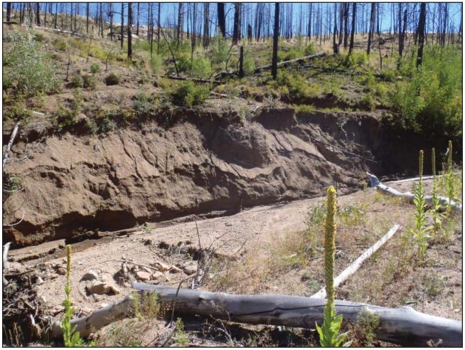
**Figure 134.** An actively eroding alluvial fan that can be restored by rebuilding the fan, relocating the channel and constructing a bankfull bench with toe wood structures.
