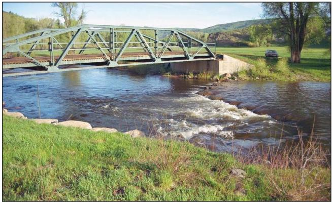
Figure 12. A rock cross-vane at a bridge crossing on the mainstem Little Snake River, Colorado.
