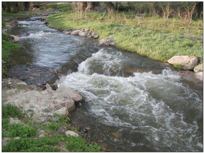
Figure 18. The "Rock & Roll" log structure implemented on the Roaring Fork of the Little Snake River, Colorado.
