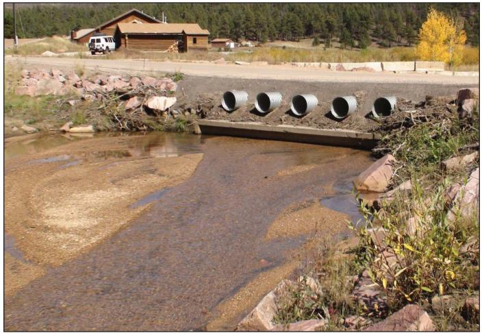
Figure 58. The aggrading box culvert (6 ft x 20 ft) and the 12" culverts on the West Creek road (looking downstream).
